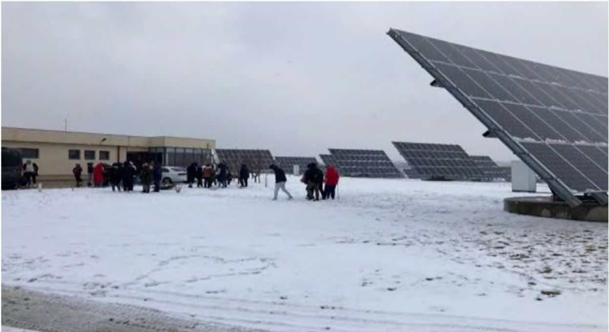
A visit to the solar farm in Miroslava
