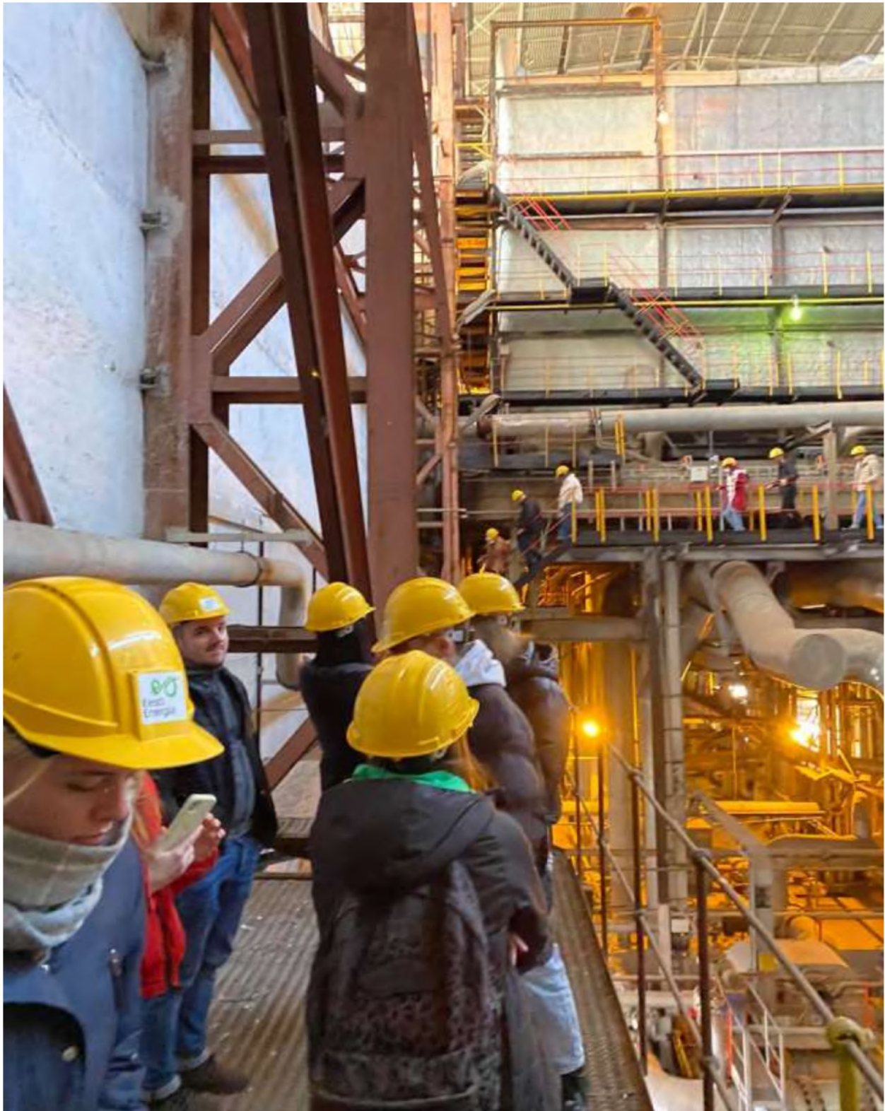
Iru Power Plant (waste-to-energy)
